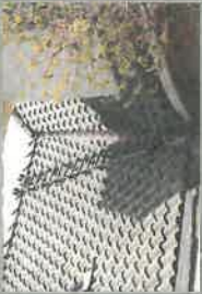
New copper valley flashing and tile roof repair. (Chicago, IL)
