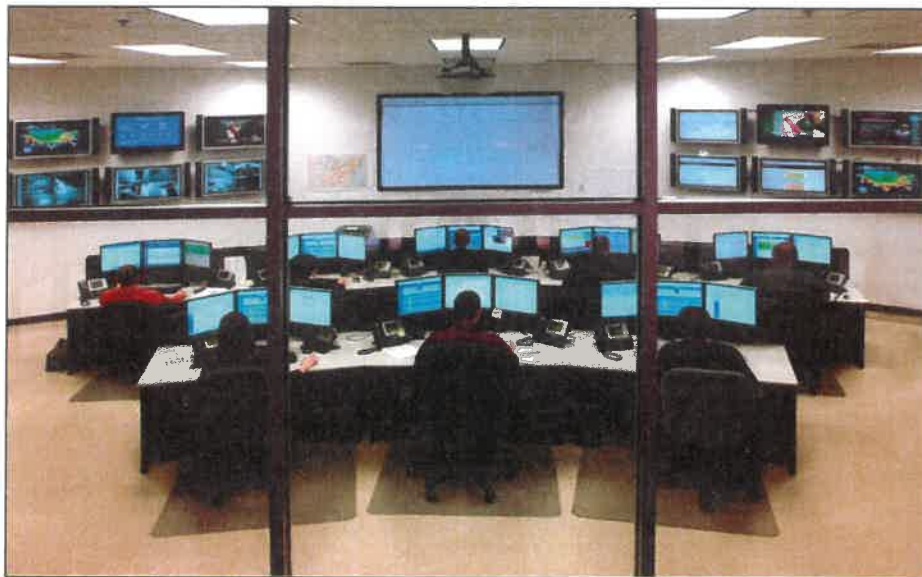
MetroNet Network Operations Center
